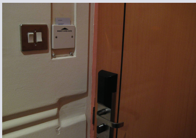
A card control located adjacent to the entrance door
