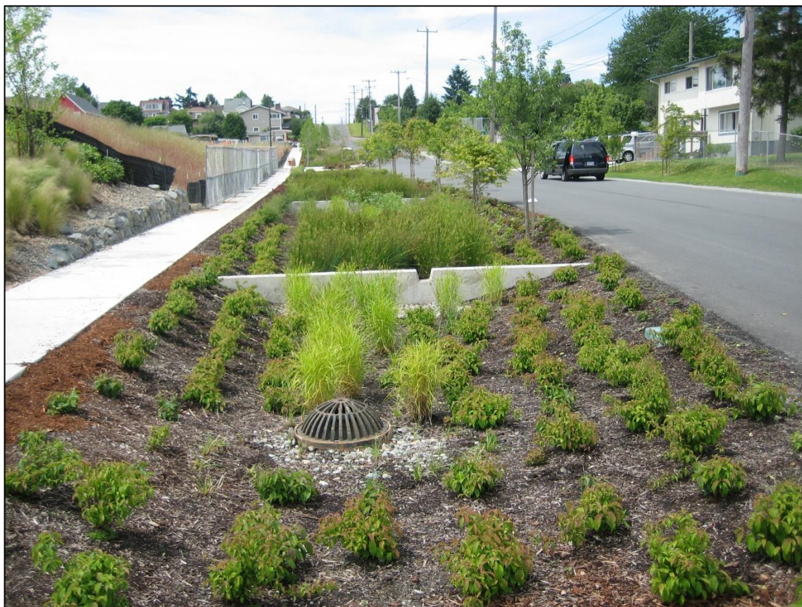
Figure 0-7— Swales with Check Dam and Overflow Arrangement (Blankenship, n.d.)
