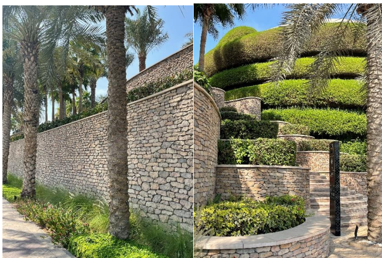
Figure 0-8— Pictures of Retaining Wall
