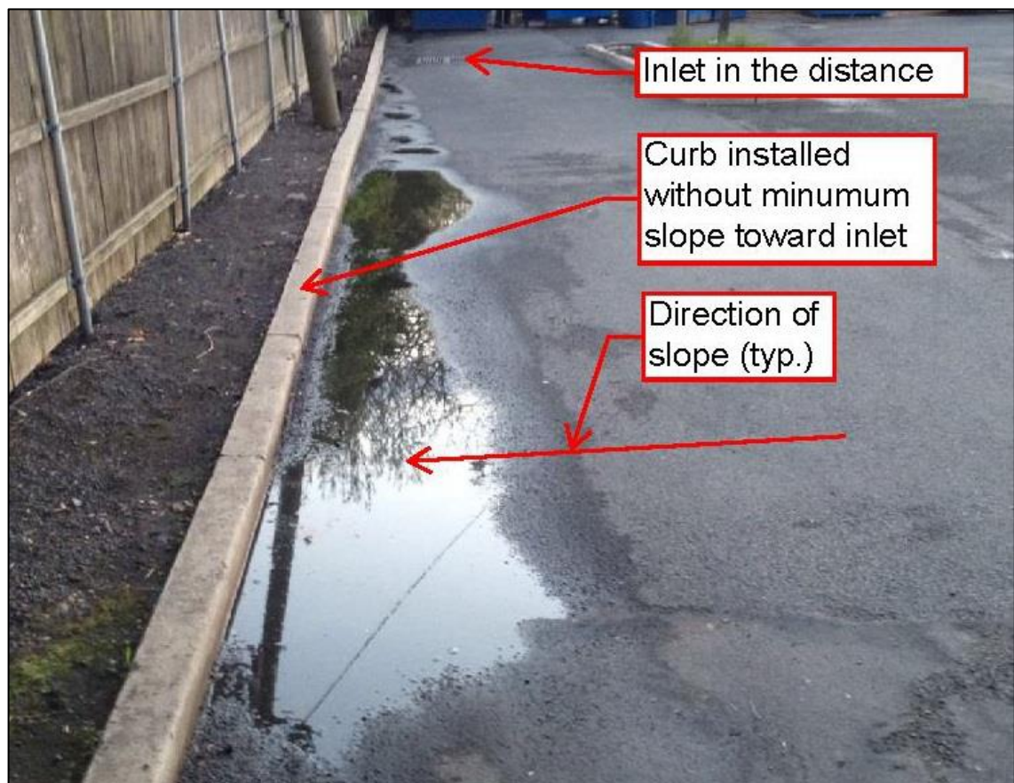
Figure 0-2— Picture of Curb Installed without Minimum Slope (Tiner, 2014)
