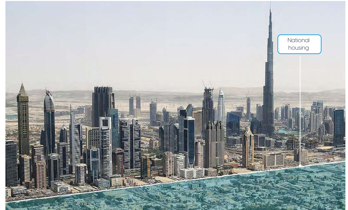
High-rise towers in DIFC overlooking National Housing across the E11 in Al Satwa
