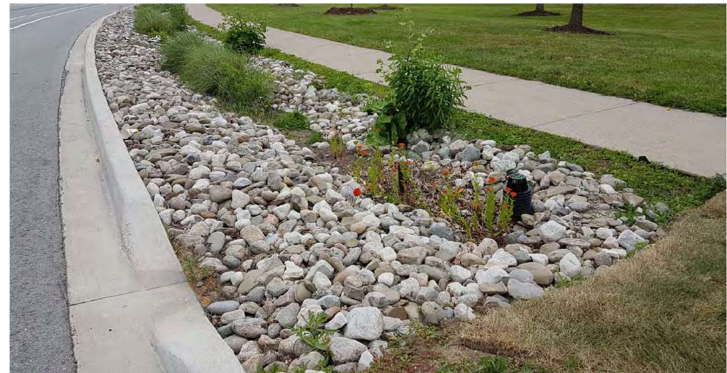
Bioswales alongside a road
