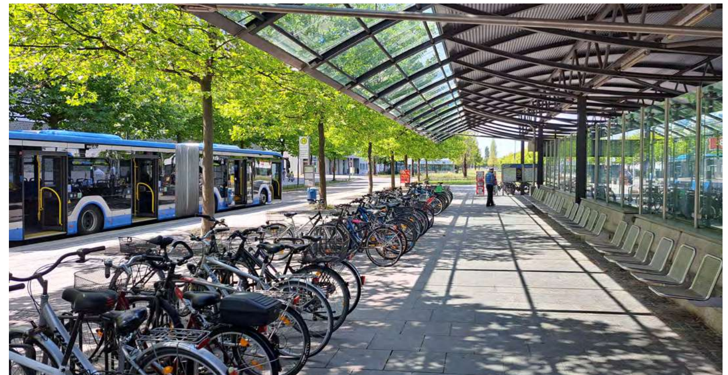
Easy and convenient multi-modal transition outside a metro station, Munich, Germany
